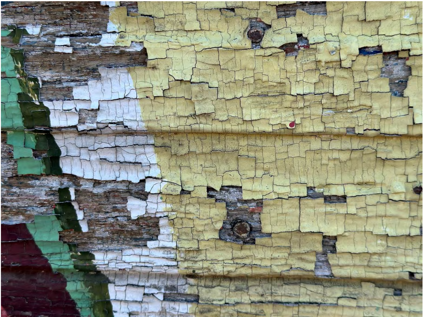
Close up View of Paint and Hardware
