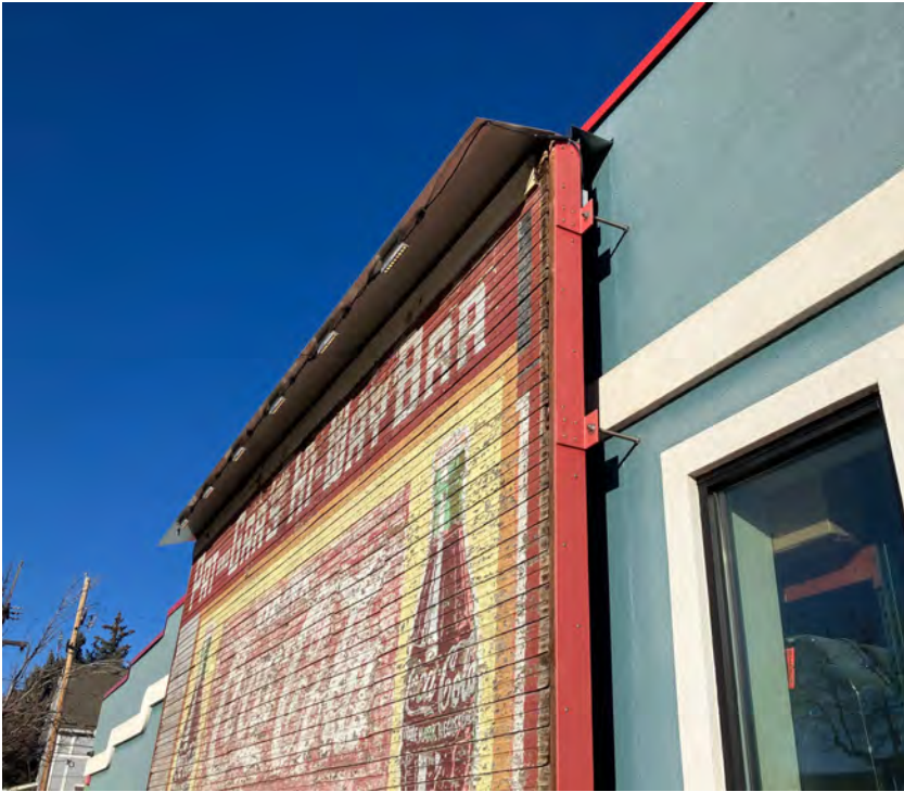
Detail of the sign structure top and east edge.
